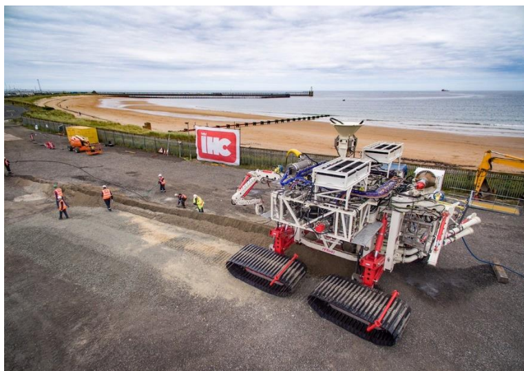
Figure 7 Aratellus Leviathan Mechanical Trencher
